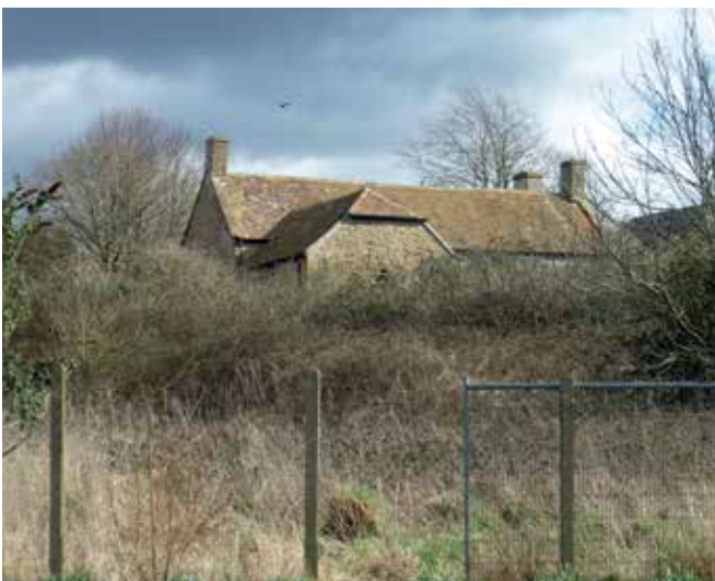
The brownfield site at Hillcrest School
