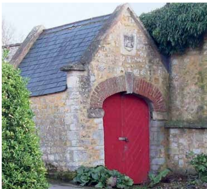
The Old Fire Station
