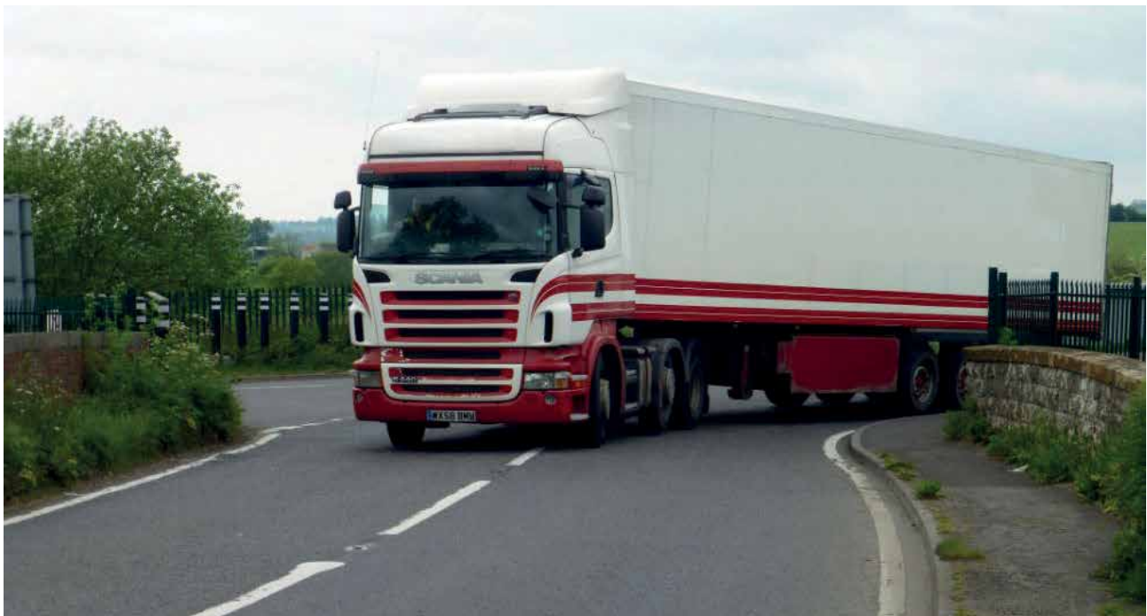
Dangerous bend on the A371 Ansford railway bridge
